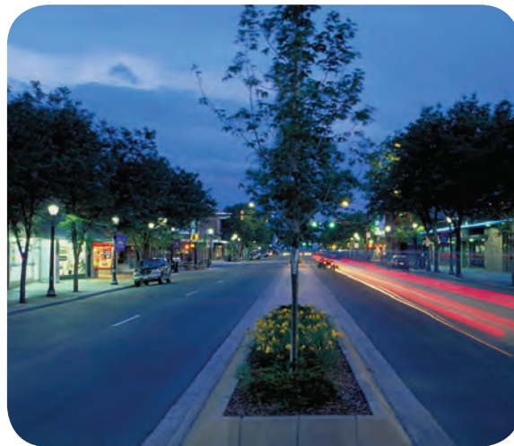
A boulevard design reduces the impact of a wide vehicular right-of-way on adjacent development.
