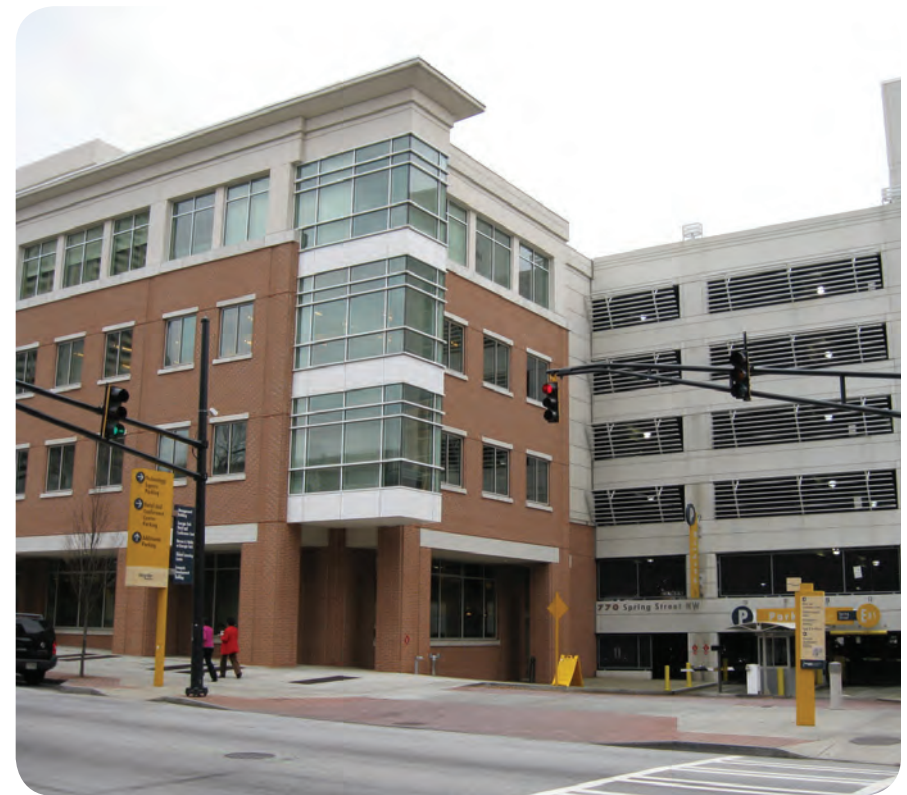
Development wrapping a parking deck is an effective way to engage parking with the building and hide it from the street.
