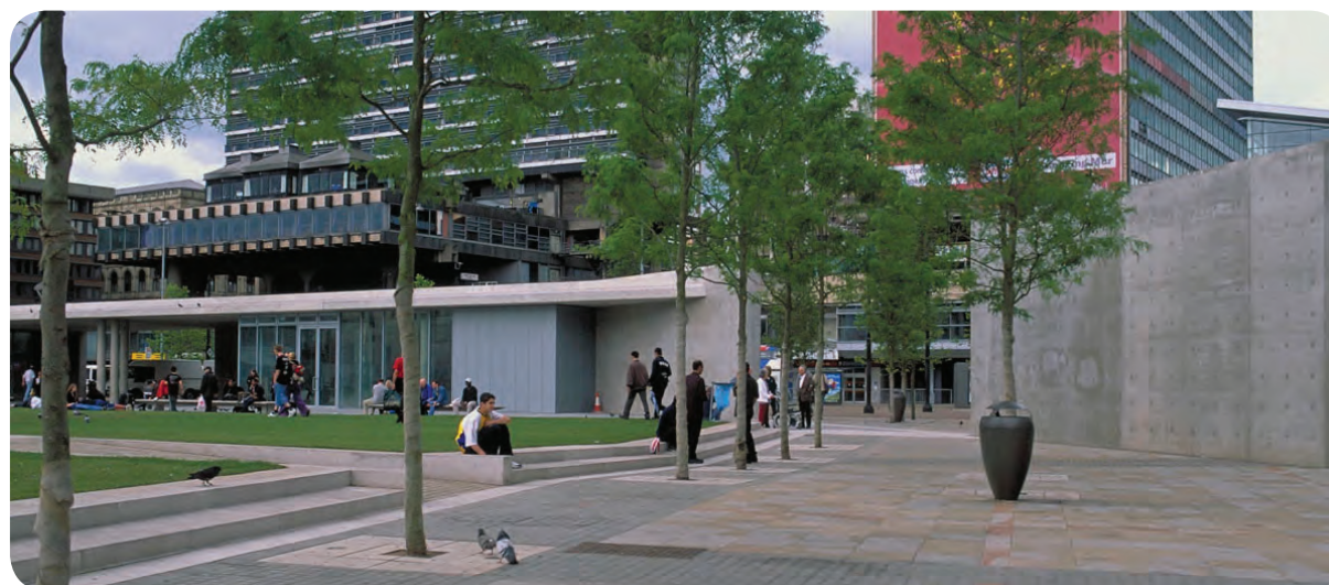
Plazas in front of station entrances enhance its civic character and make transit a focal point. (Manchester, England)
