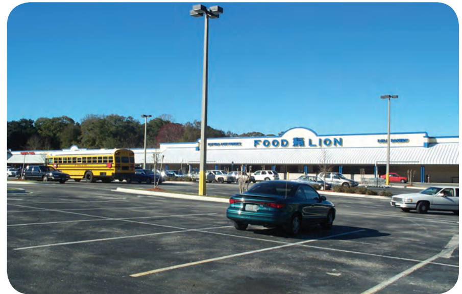
Building is significantly disengaged from the street thereby eliminating any consideration for a pedestrian oriented environment
