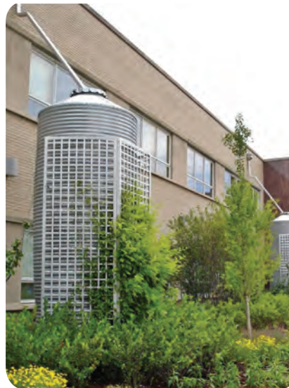
This cistern (above left) collects rainwater and stores for irrigation. The planting strip along this street is a 'rain garden' (above right) that filters stormwater runoff and recharges the water table, reducing the treatment costs for the City.
